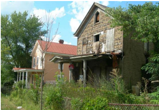
1326 Valley Place SE, showing demolition by neglect, and the adjacent house at 1320, restored with a historic homeowner grant
