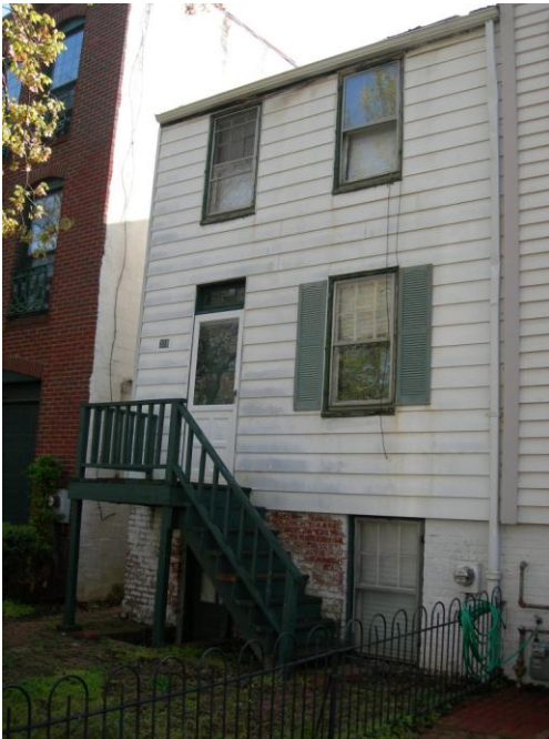
308 9 th Street in April 2009, before renovation
