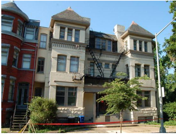
1841 16 th Street NW in June 2008, before stabilization
