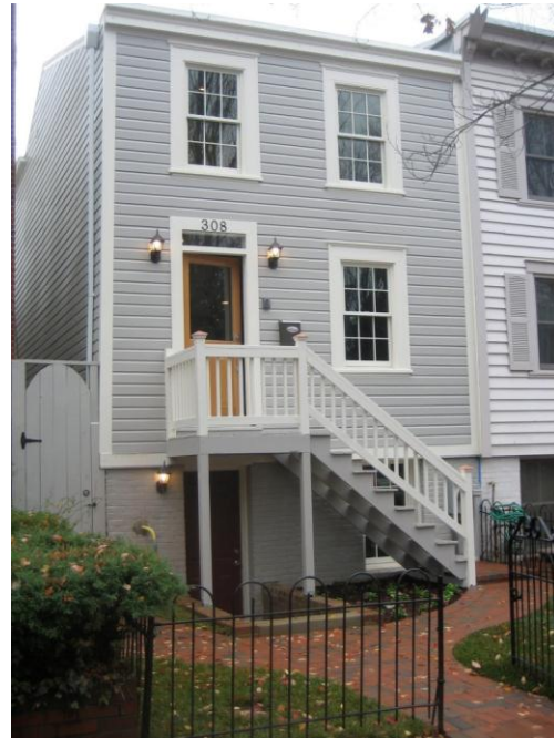
308 9 th Street after being placed back into service
