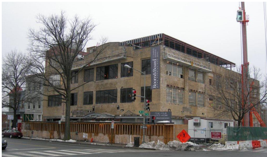
Room & Board under construction at 14 th and T Streets, NW
