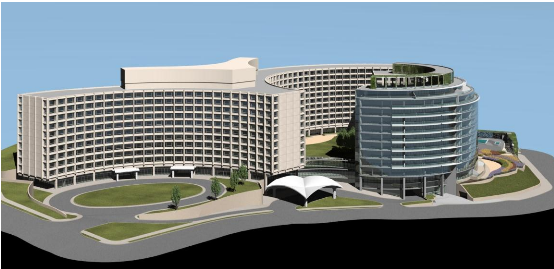
Washington Hilton renovation and addition (courtesy Beyer Blinder Belle Architects & Planners)
