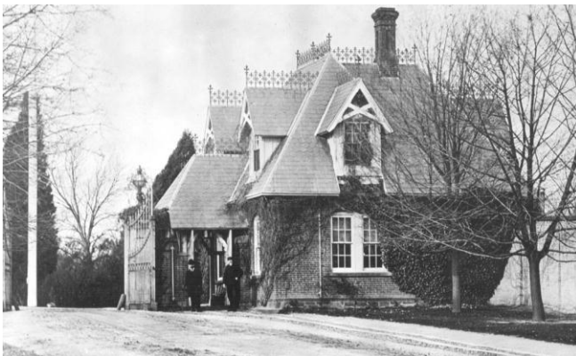
The Victorian gatehouse at the main entrance to the West Campus of Saint Elizabeths Hospital will be restored to its historic appearance as part of the perimeter security project for the new Department of Homeland Security headquarters
