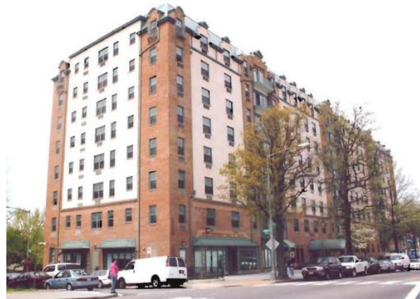
Cavalier Apartments after completion
