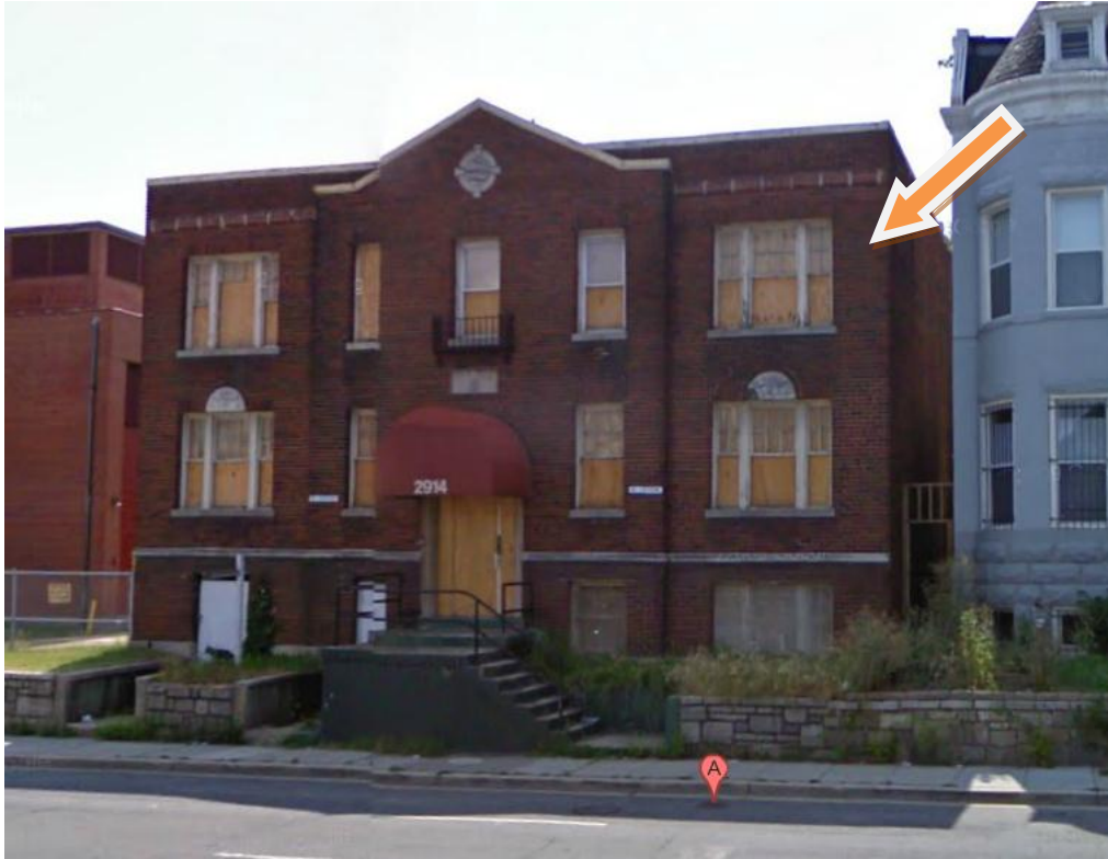
Figure 2: Front of Subject Property
