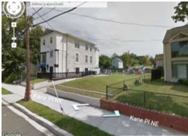
Side of Building
