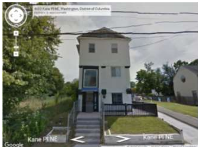
Front of Building
