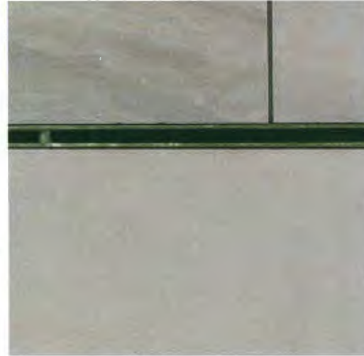
ADA COMPLIANT METAL RUNNEL
