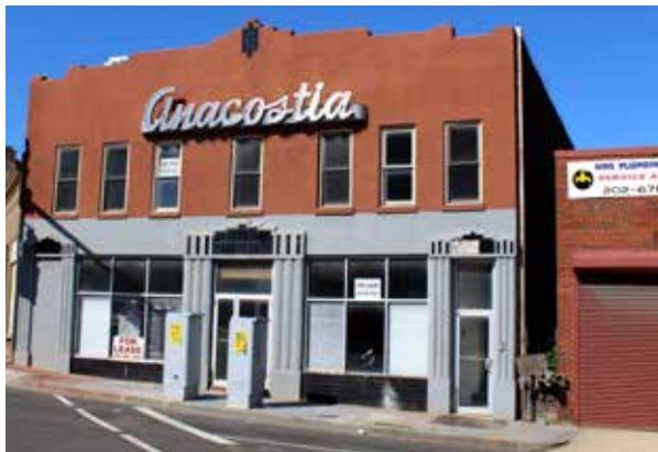
Commercial buildings in the Anacostia Historic District
