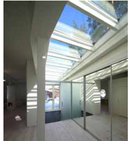
Skylights can boost energy efficiency by bringing natural light to the interior of long rowhouse units with no side windows
