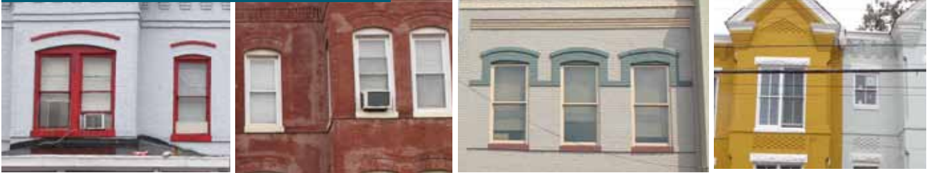
Typical window configurations. Paired windows may sit in a single opening with brick detailing above or below
