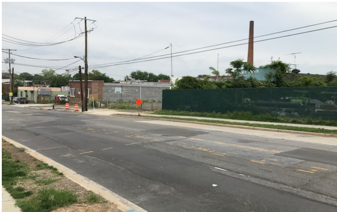
Photo 2 - View facing front corner of existing property - inbound
