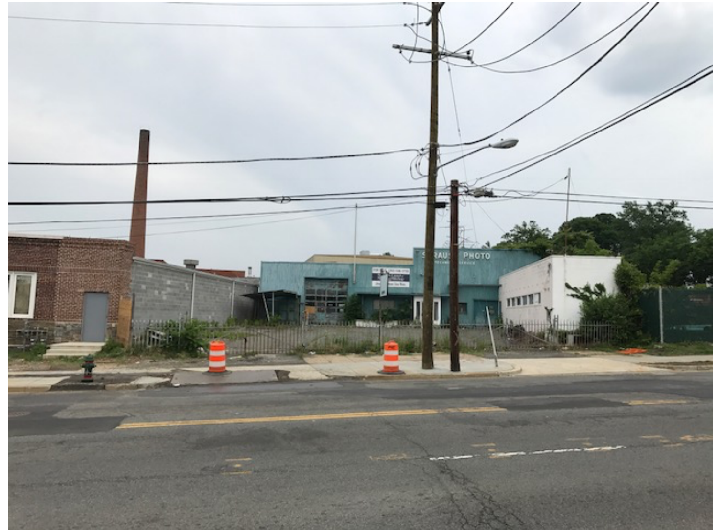
Photo 3 - View facing front of existing property
