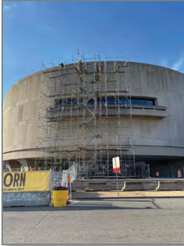
Hirshhorn Museum re-cladding
