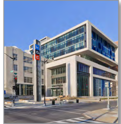
Compatible additions to historic landmarks: NPR Headquarters building
