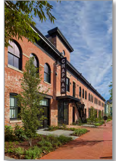
Adaptive reuse of the historic Chapman Coal Company Garage and Stables for housing
