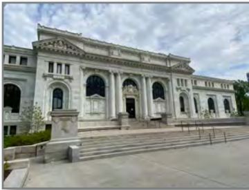
Preservation of District-owned properties, Franklin School and Central Library
