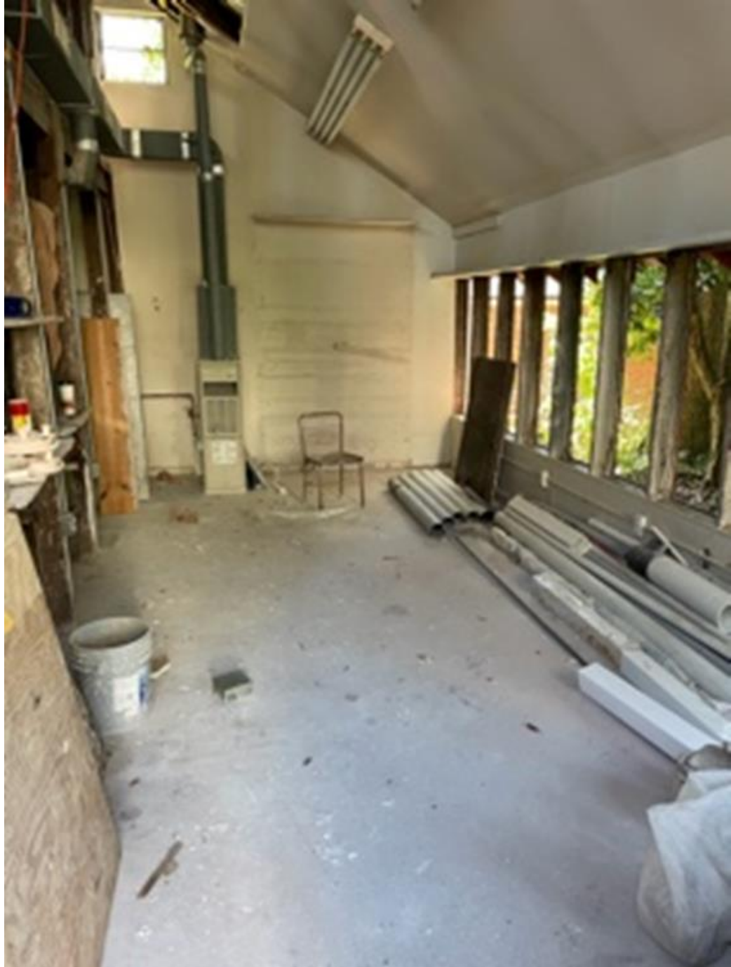
Modern concrete floor and foundation of 515 Cedar outbuilding
