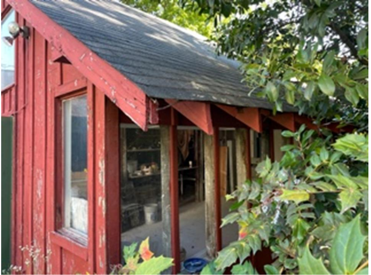
Modern roof framing and plexiglass windows at 515 Cedar outbuilding
