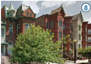
⑧ The northern edge condition is of a primarily residential typology, lending itself to a more quiet setting.
