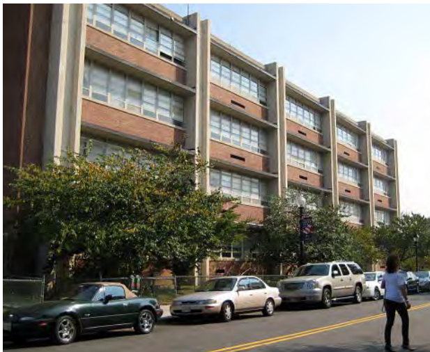
Hine Junior High School, built in 1966 and operated until closed in 2008; since then adapted into a mixed-use development
