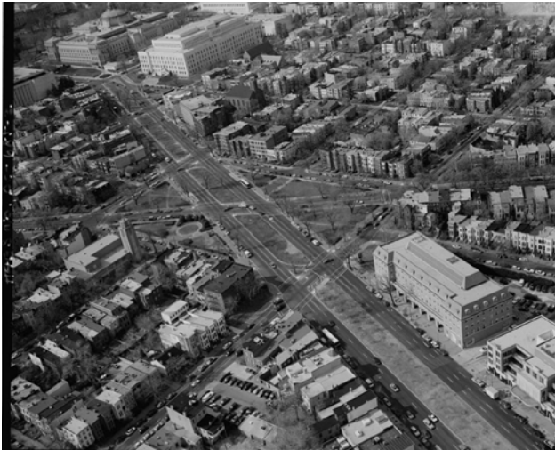
An aerial view of Seward Square looking Northwest along Pennsylvania Avenue SE - photo taken from the HABS DC-685 survey
