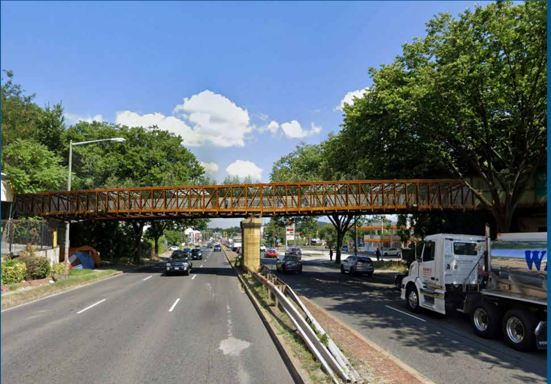
Rendering of Ivy City pedestrian bridge crossing New York Avenue NE facing east. The bridge is constructed out of a reused railroad bridge, preserving its industrial architecture and creating a safer pedestrian crossing.
