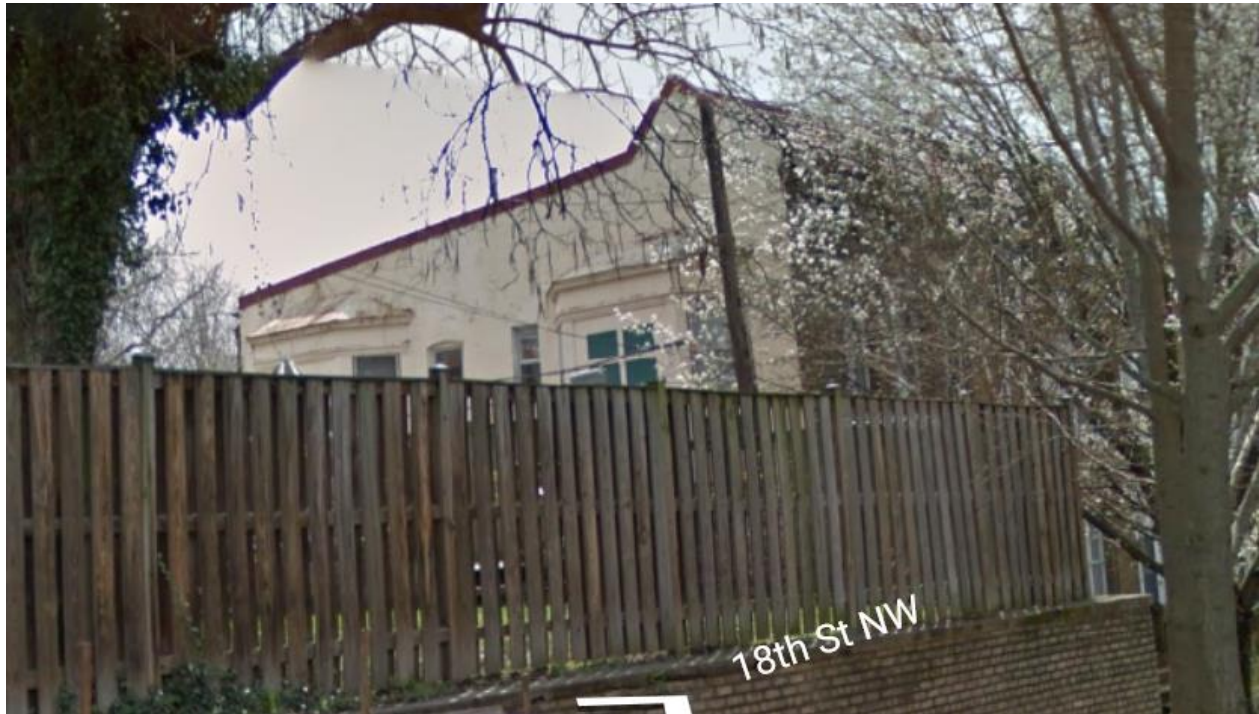
A Google Streetview image of the side of the building in April 2014.
