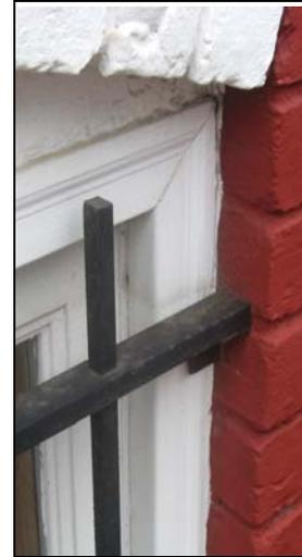
*Original rounded brick molding (left); flat replacement molding does not replicate the original profile (right).*
