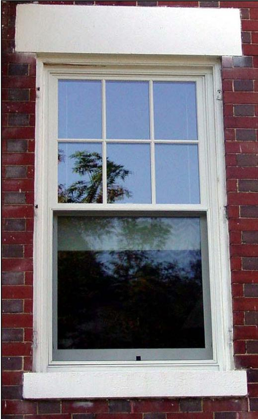
*The muntins and exterior framing elements on these replacement windows (above and below) replicate the profiles of the original windows.*
