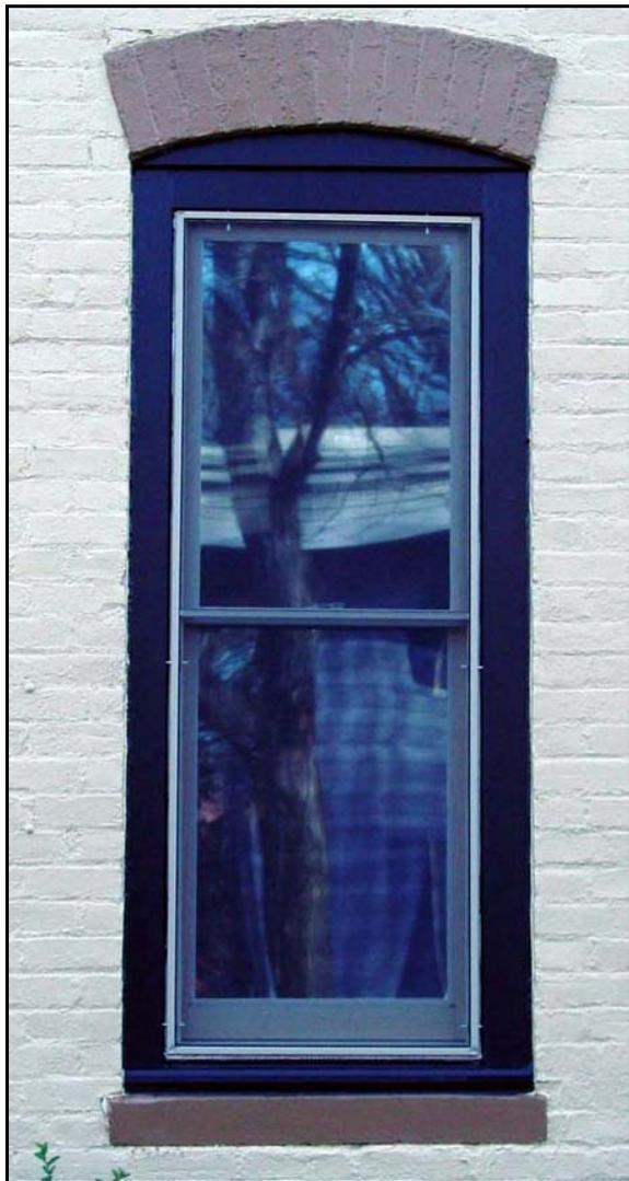
*This pocket window replacement (above) has noticeably thicker framing and less glass than the original window (right).*
