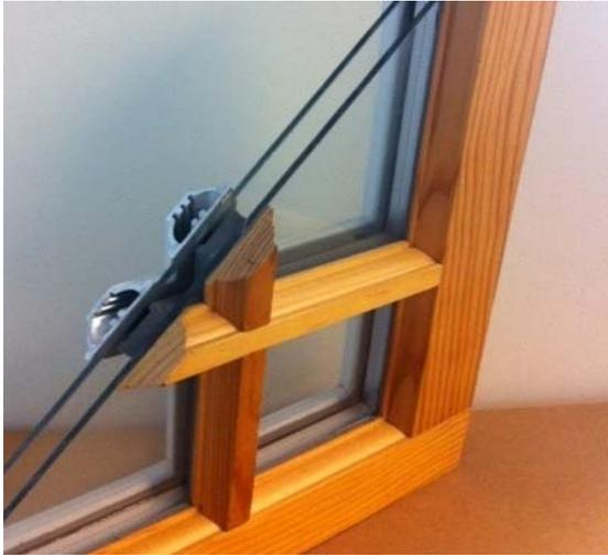
*This cut-away section of a simulated divided light window has an interior and exterior muntin with a beveled profile that replicates the appearance of an historic window.*
