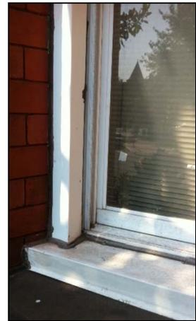
*Original rounded brick molding (left); aluminum capping covers and flattens the original profile (right).*
