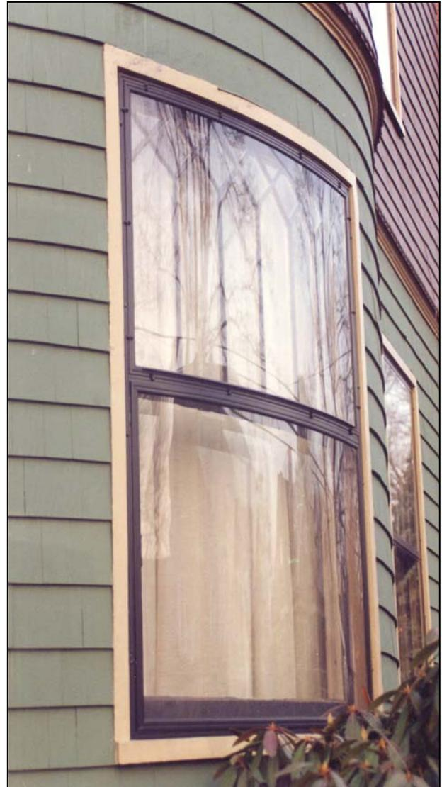
*This storm window was fabricated to preserve and improve the energy efficiency of a special curved glass window.*
