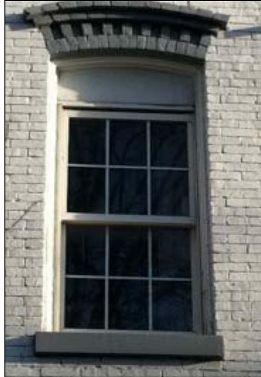
*This replacement window does not properly fit the original opening.*
