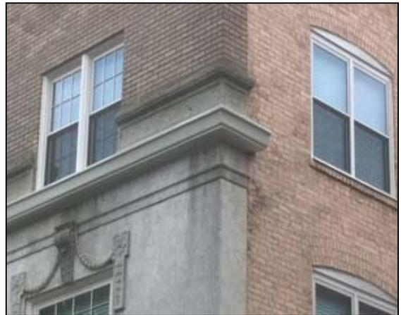
*The replacement windows on the primary elevation (at left) closely match the original appearance. The windows on the secondary elevation (at right) fit their openings and match the general character of the original windows.*
