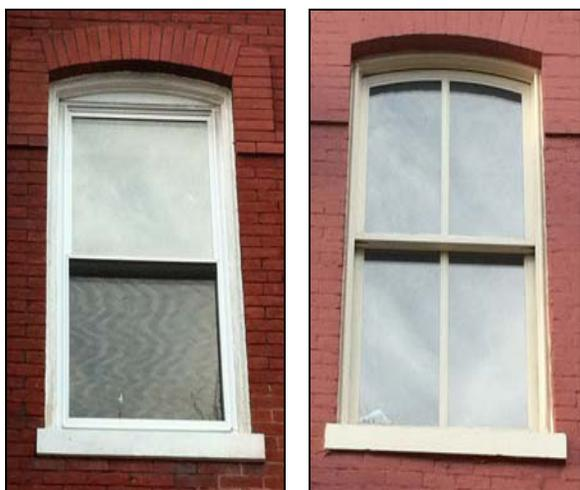
*These new windows (at left) do not replicate the profiles, dimensions, fit or visual appearance of the originals (right).*
