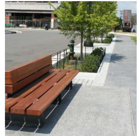
Bioretention tree pits help manage stormwater runoff.
