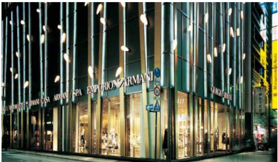
Internally lit show windows and incorporating lights into the façade of a building can add secondary light in a way that complements neighboring buildings and public space.
