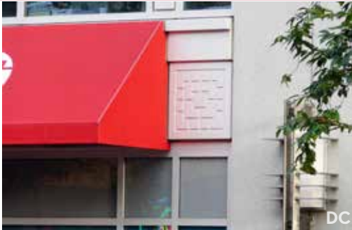
Decorative patterned motif inset into precast concrete panels
