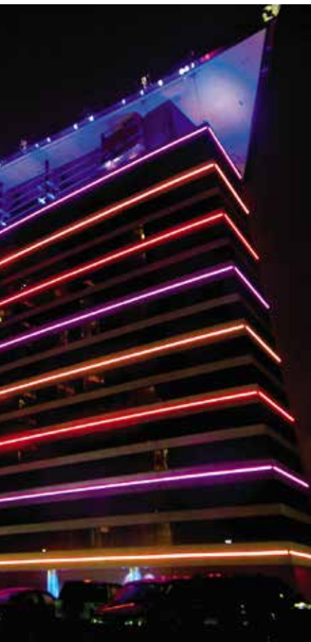
Decorative Contemporary Exterior Lighting effects can contribute greatly to the identity of Chinatown.
