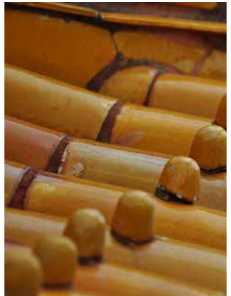
Terra cotta is an iconic Chinese building material used in awnings and roofs.
