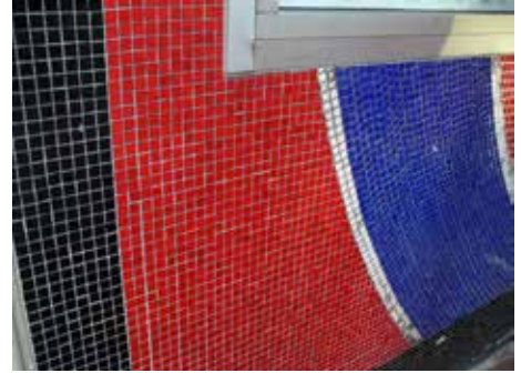
Ceramic tiles are a flexible building material that can be used to create intensely colored façades.
