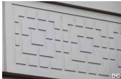
Decorative patterned motif inset into precast concrete panels
