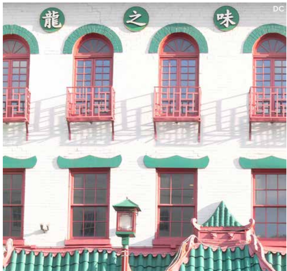
Color and the design of the entire window opening and surround can be used to include Chinese symbols and elements such as railings and medallions.
