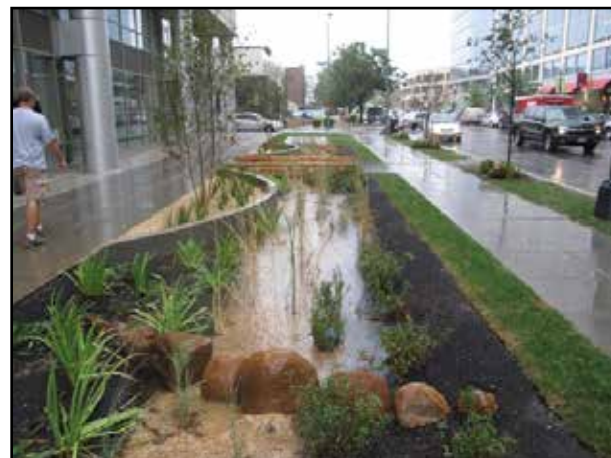
1200 First Street, NE, rain garden on a rainy day
