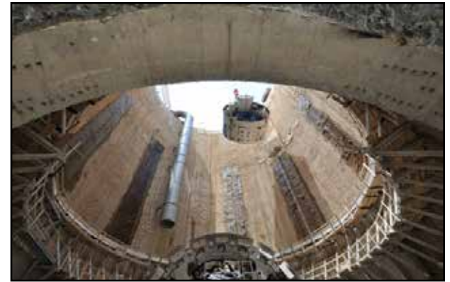
The "Lady Bird" tunnel boring machine being lowered into a shaft at Blue Plains
