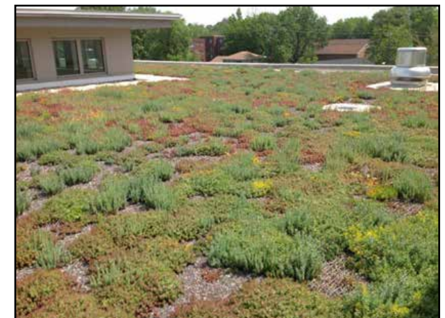
Green roof at Woodson High School, funded by ARRA
