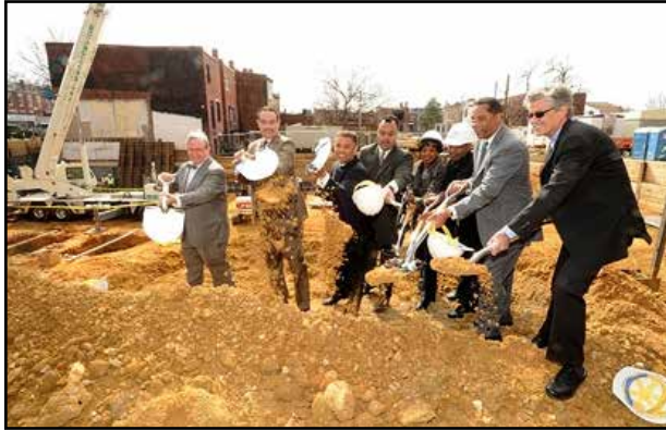
The Heights at Georgia Avenue Groundbreaking (FY 12)
