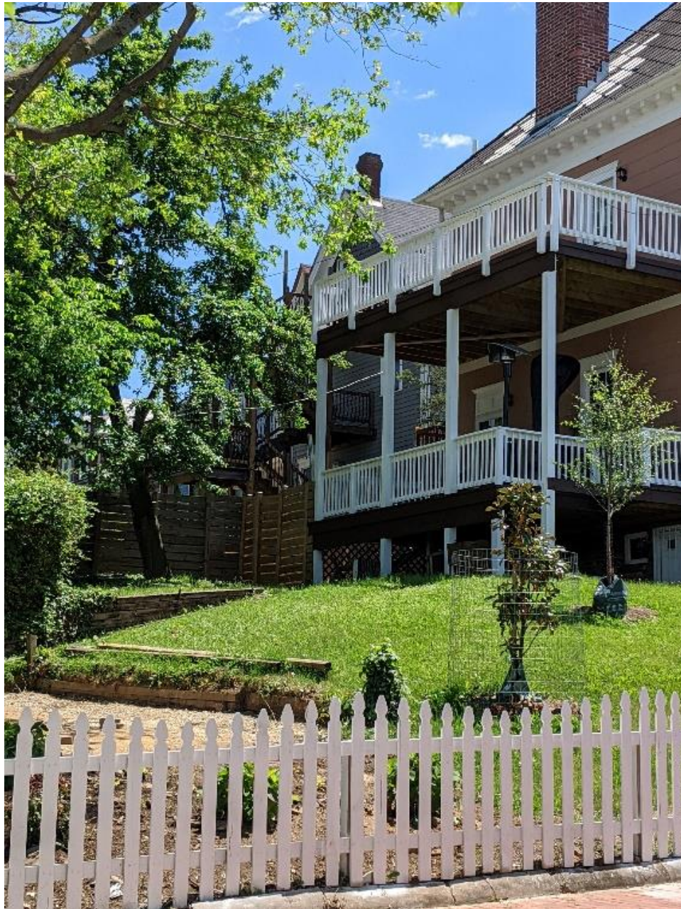
Completed Rear Staircase and Deck from Chester Street
