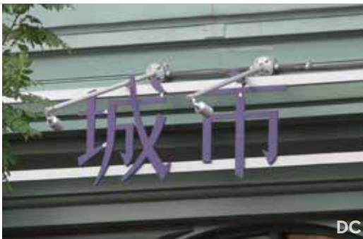
Chinese characters pin-mounted to building façade
