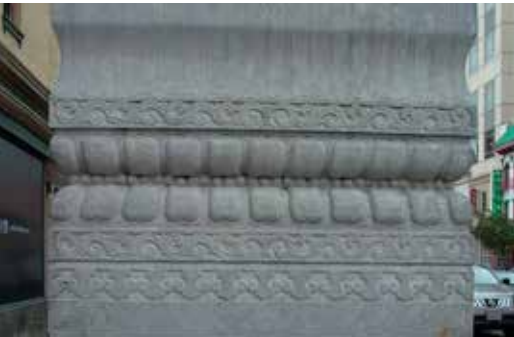
Traditional decorative motif in precast at roof line
