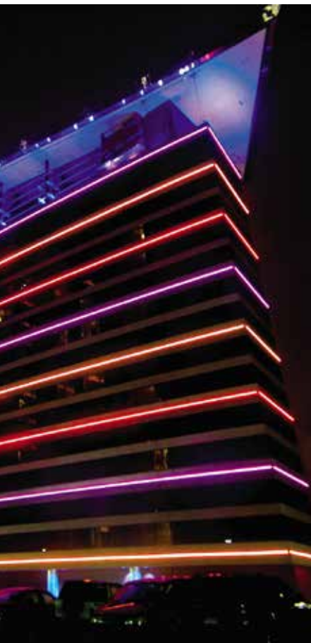
Decorative Contemporary Exterior Lighting effects can contribute greatly to the identity of Chinatown.
