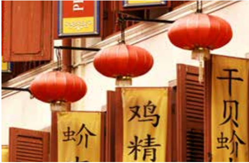
Creative integration of brackets and Chinese lanterns on building façade
