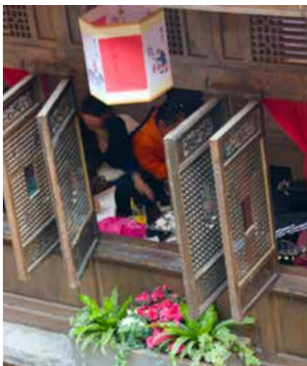
Open windows at the ground level create an appealing relationship to the street.
