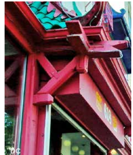
Elements that support awnings are also important for defining Chinese character.
