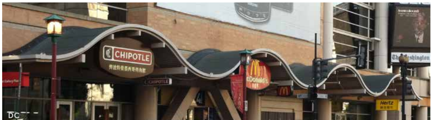
Modern and contemporary awnings can be iconic building features that evoke traditional Chinese building principles.
