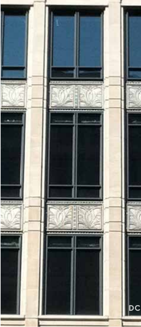
Details on upper façades should be bold so that they are easily seen from the street.
