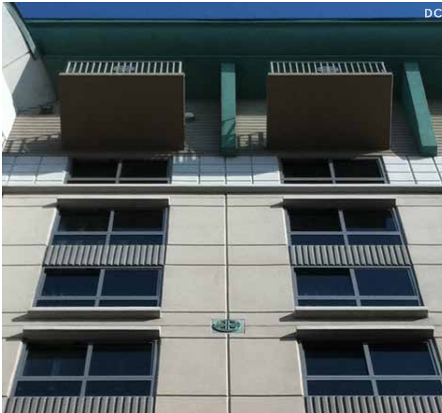
Windows can be spaced to allow room for Chinese details on the upper floors of a building façade.
