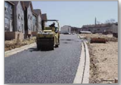
Housing construction at Wheeler Creek in the Congress Heights neighborhood
