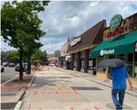
7 Temporary pedestrian-only path outside of storefronts
