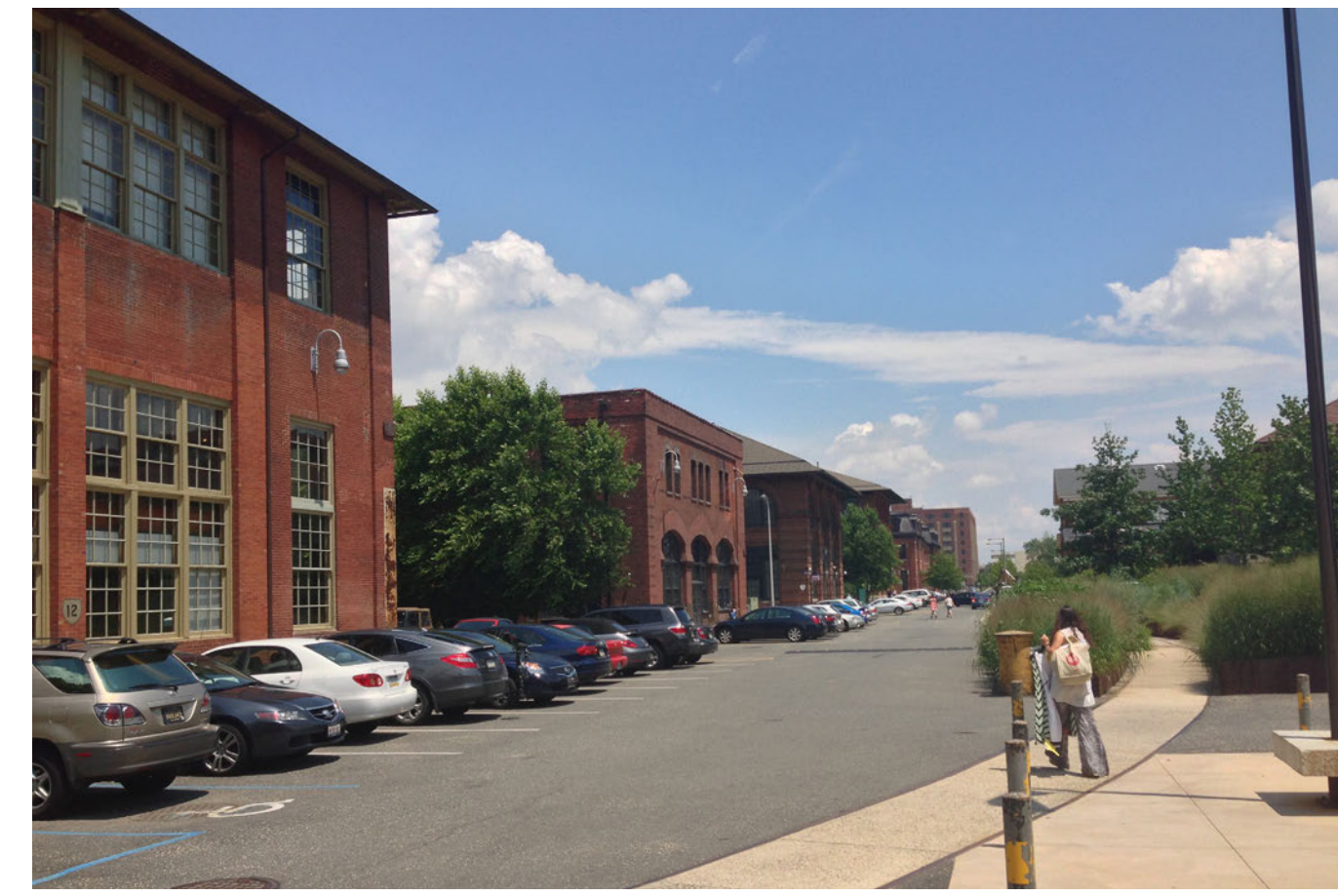
Adaptive Reuse of Historic Structures, The Navy Yard, Philadelphia.
