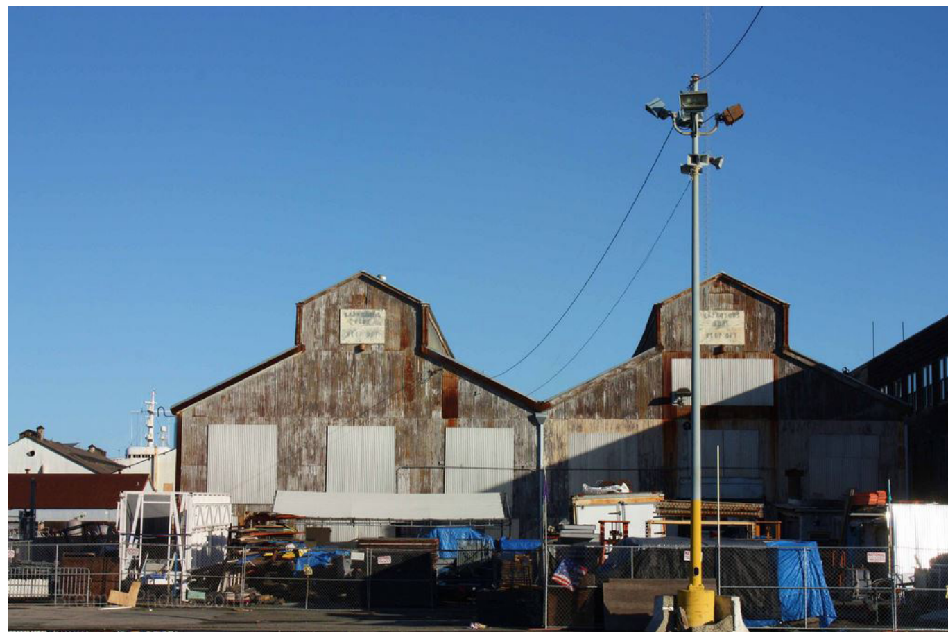
Pier 70 in San Francisco.
