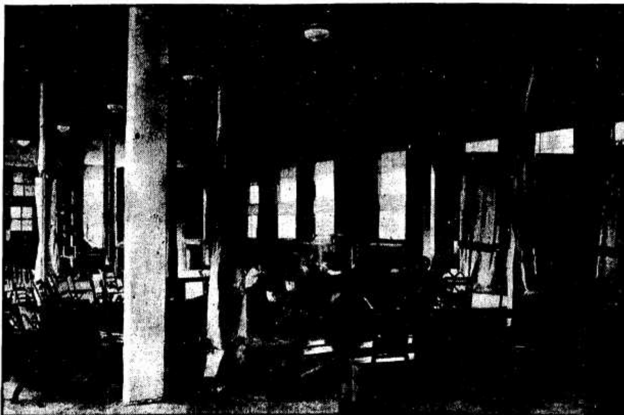
This unfinished big room is the second floor of a wing at the Rose Lees Hardy School, left incomplete when the Government's economy program was launched two years ago. The class rooms on the first floor are overcrowded and this space is needed. The Board of Education has asked that it be partitioned and finished as regular rooms. The children use it now for special conferences, to plan school activities and to train for their public programs. It is the only assembly hall in the building. The project is on the list submitted for the new public works program. —Star Staff Photo.
