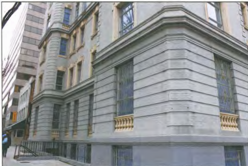
Photo #0004: DC_The Ethelhurst_0004.tif Exterior; northwest corner detail, camera facing southeast
