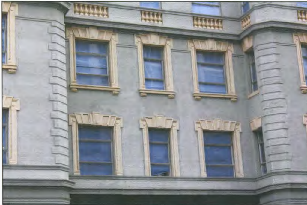
Photo #0009: DC_The Ethelhurst_0009.tif Exterior; detail of west upper windows, camera facing east
