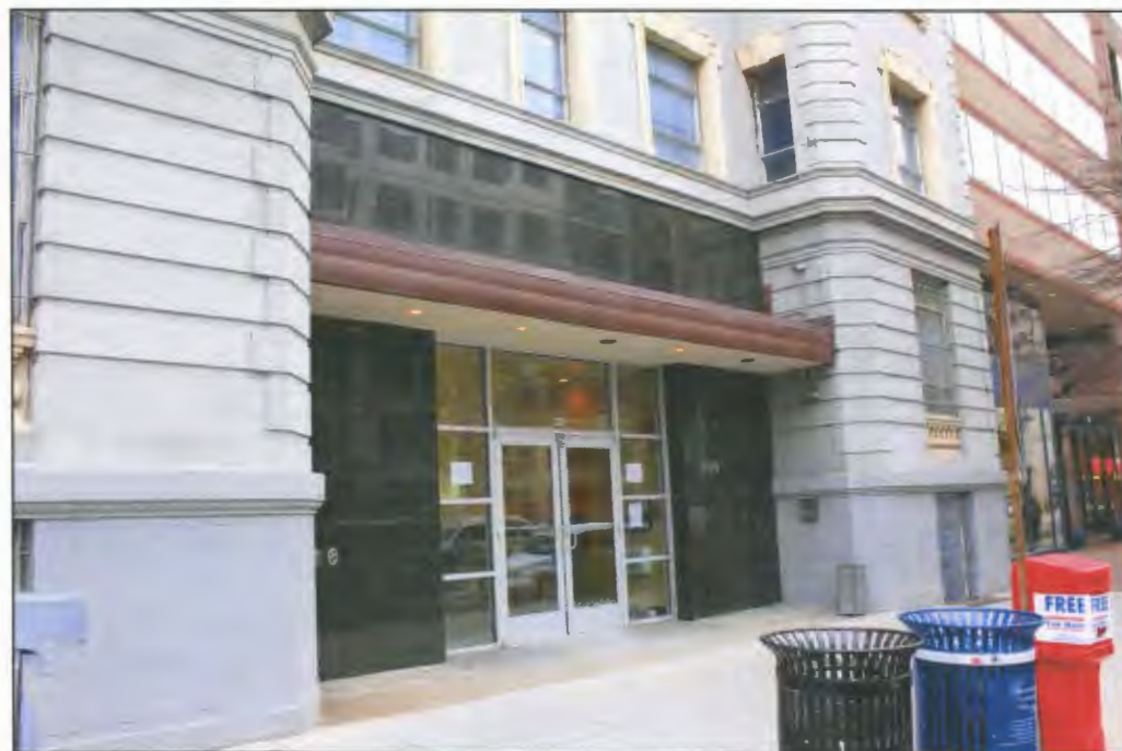
Photo #0005: DC_The Ethelhurst_0005.tif Exterior; west entrance oblique, camera facing southeast
