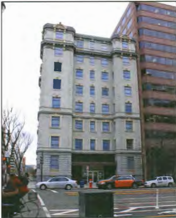
Photo #0002: DC_The Ethelhurst_0002.tif Exterior; west elevation, camera facing northeast
