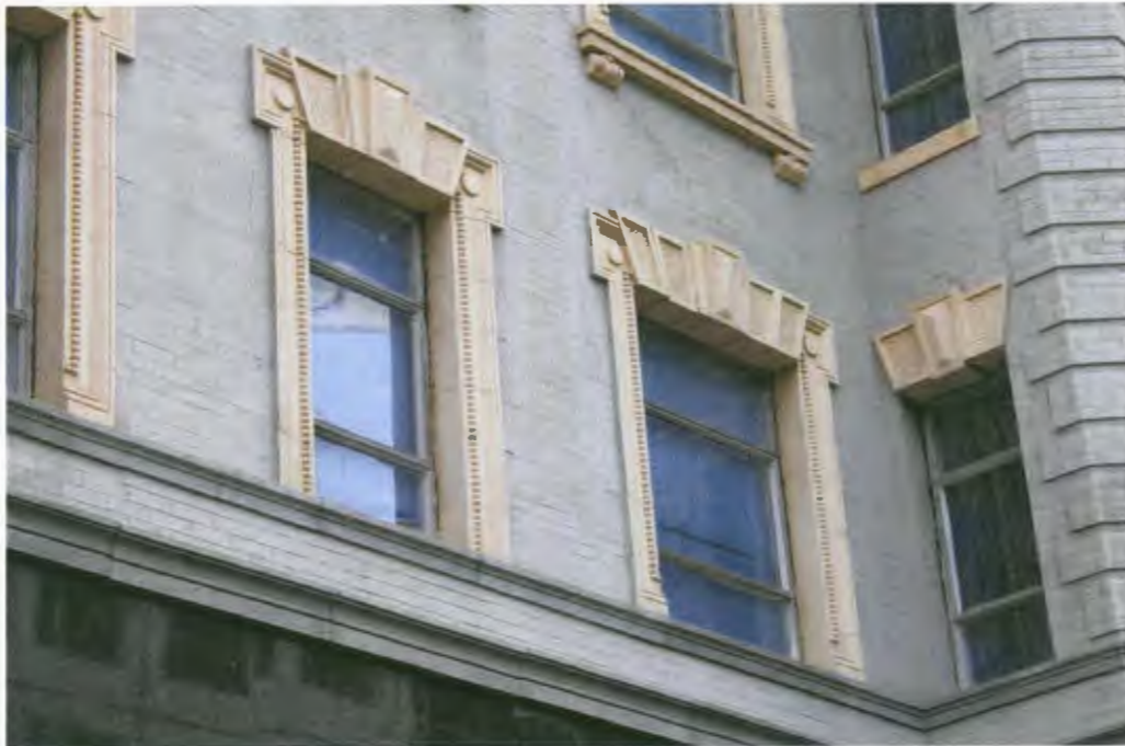
Photo #0007: DC_The Ethelhurst_0007.tif Exterior; detail of west windows, camera facing southeast
