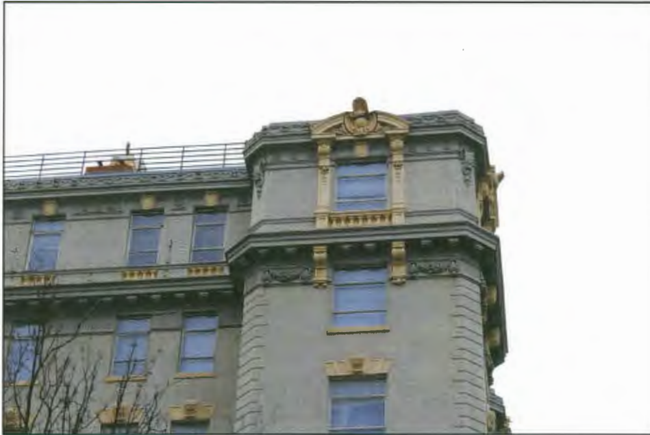
Photo #0010: DC_The Ethelhurst_0010.tif Exterior; detail of north cornice, camera facing south
