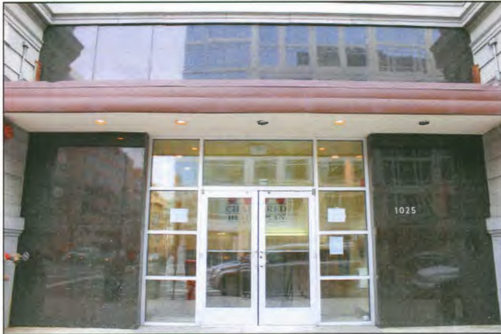
Photo #0006: DC_The Ethelhurst_0006.tif Exterior; detail of west entrance, camera facing east
