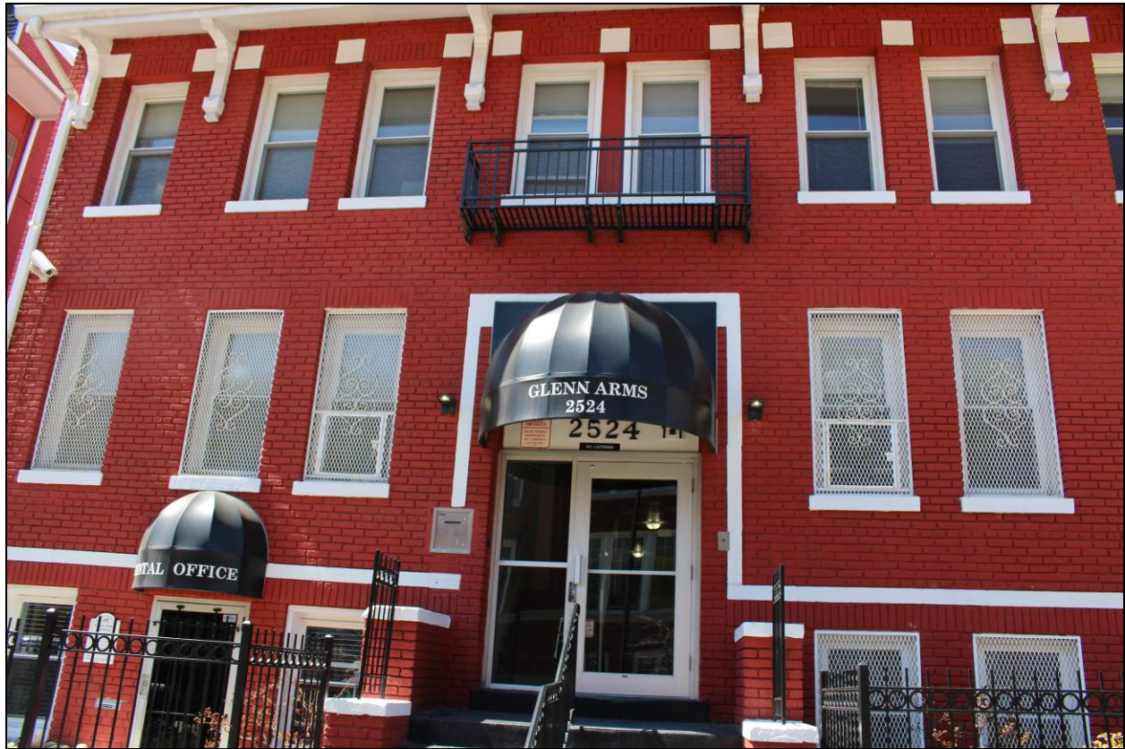
Exterior: Detail of façade, entry, looking west
