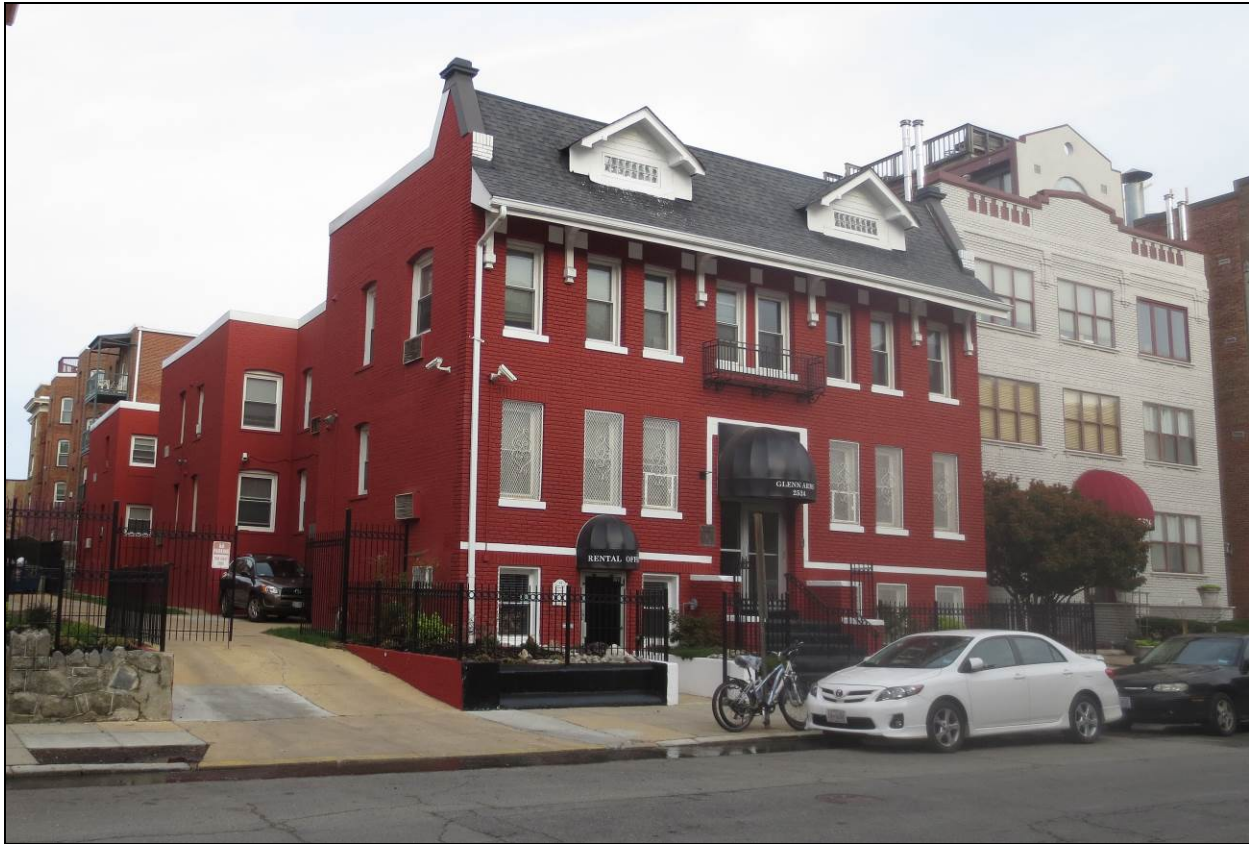
Exterior: Façade and south elevation, looking northwest
