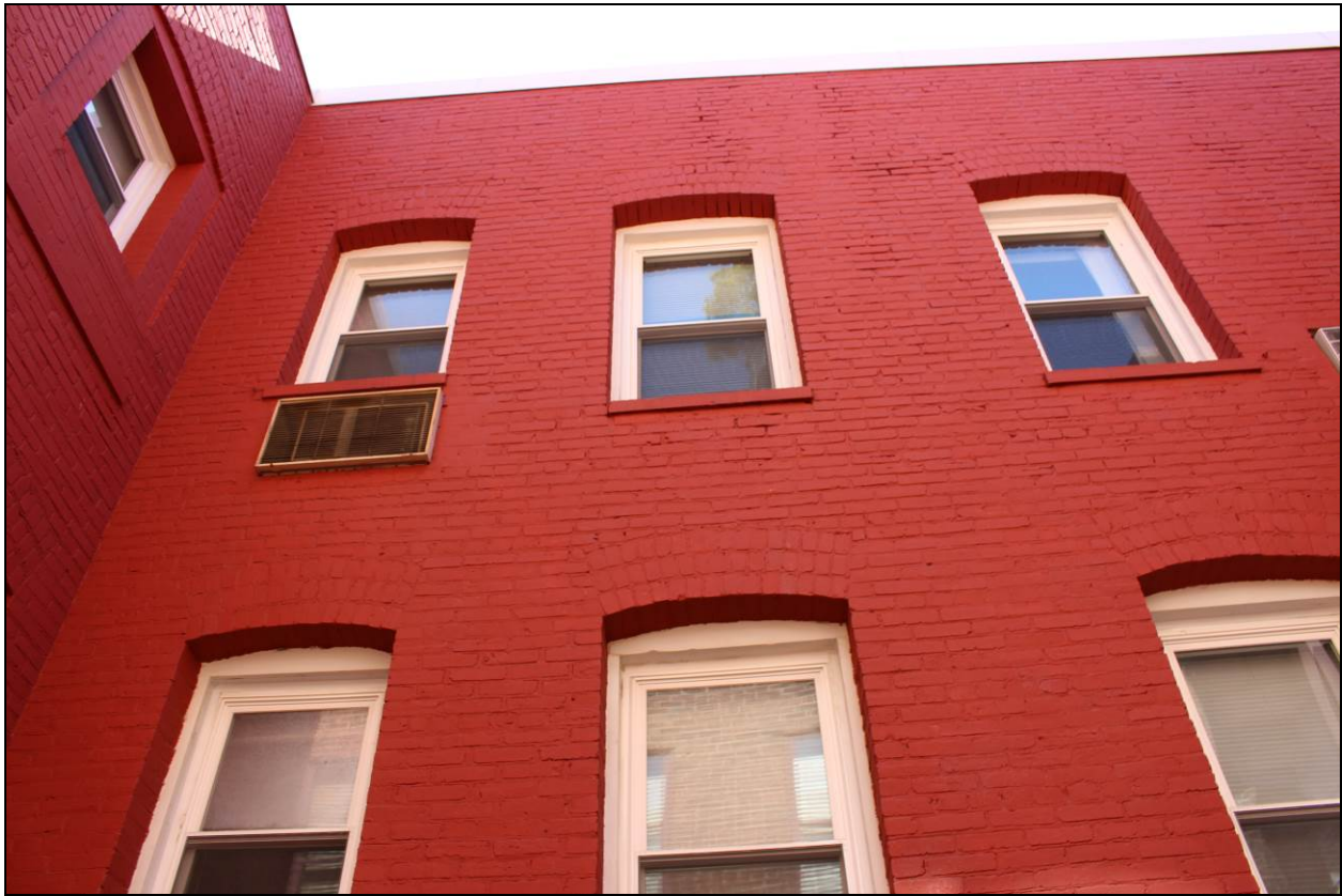
Exterior: Detail of north elevation, looking south
