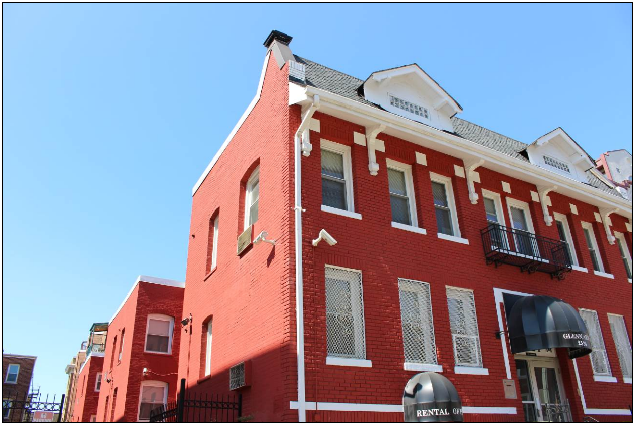
Exterior: Southeast corner, looking northwest
