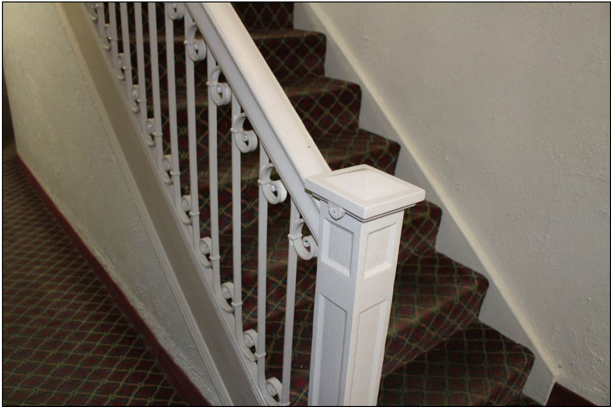
Interior: Detail of first floor stair
