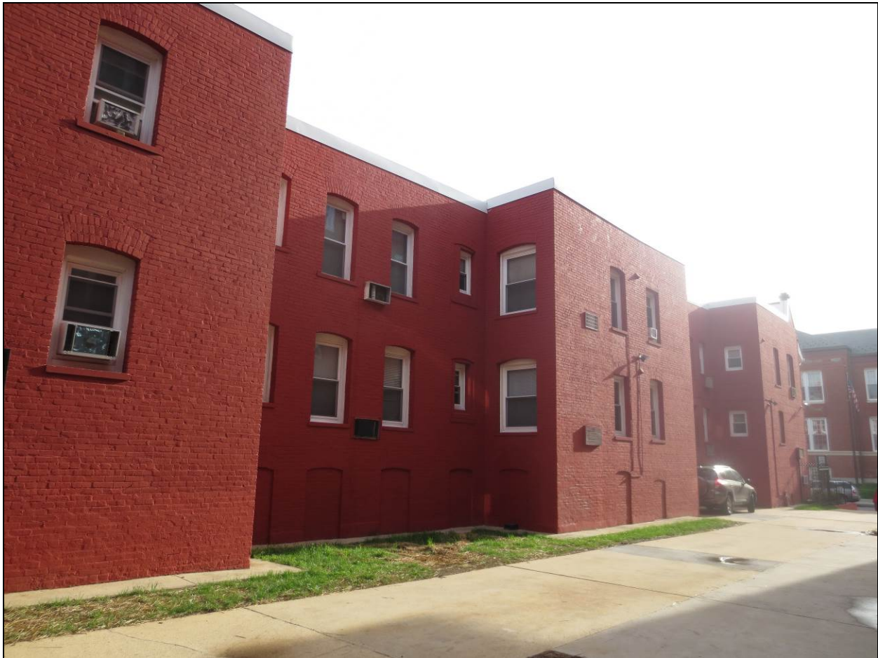
Exterior: South elevation, looking east
