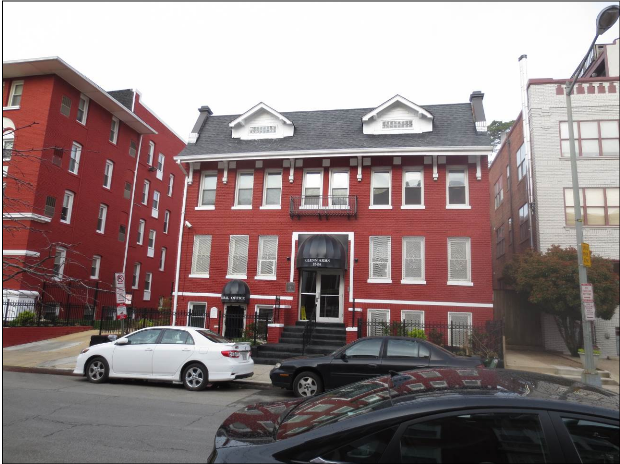
Exterior: Façade, looking southwest
