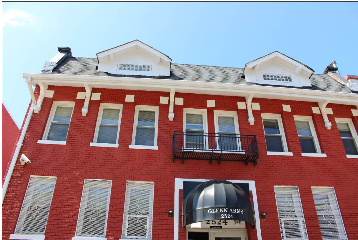
Exterior: Detail of façade, looking northwest
