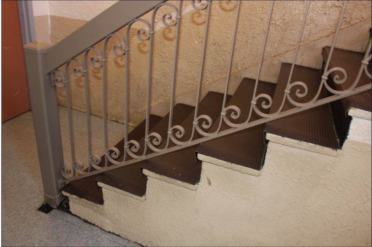
Interior: Detail of stair on first floor
