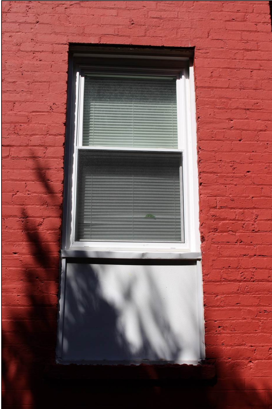
Exterior: Window detail on south elevation
