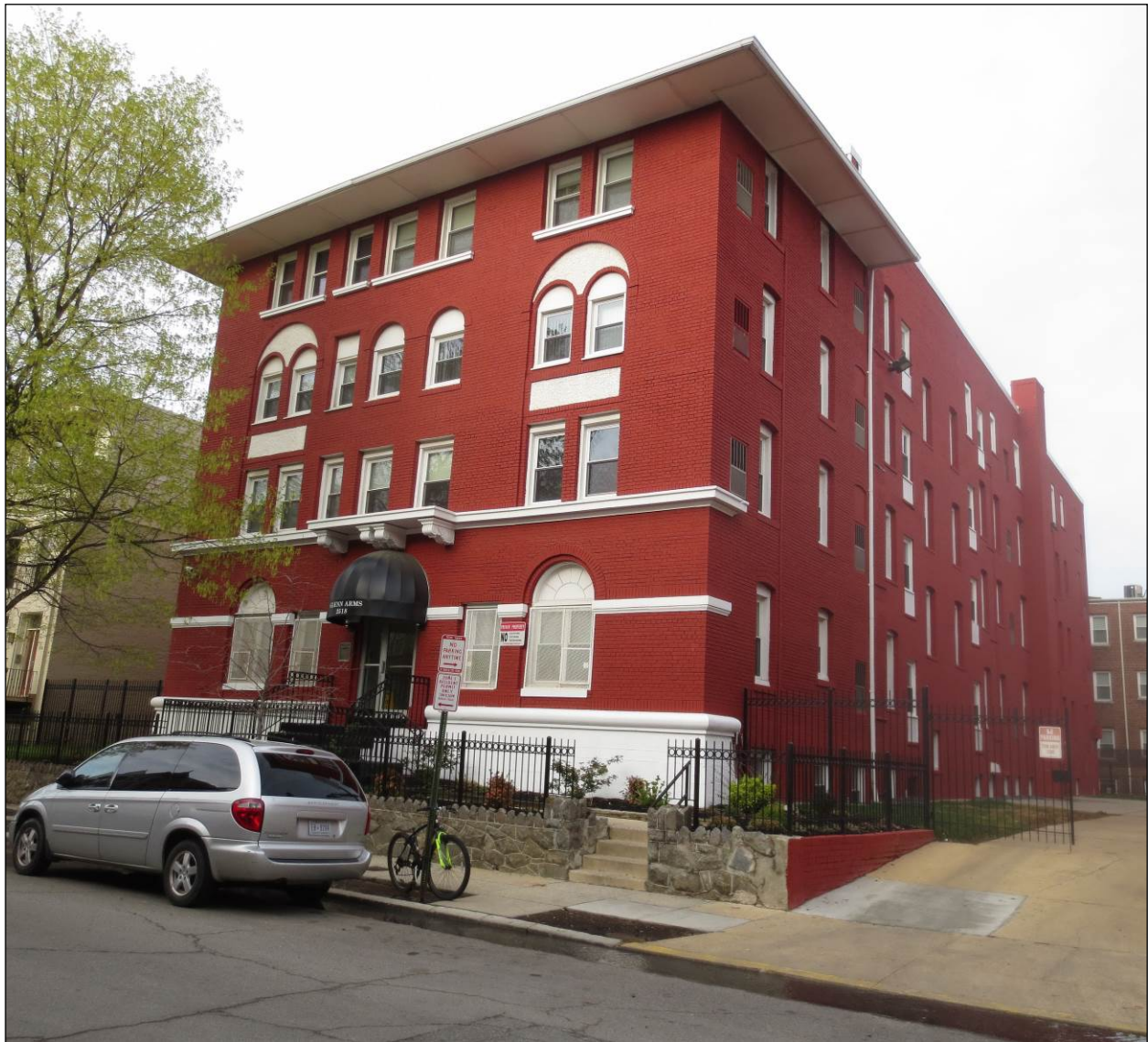
Exterior: Façade and north elevation, looking southwest
