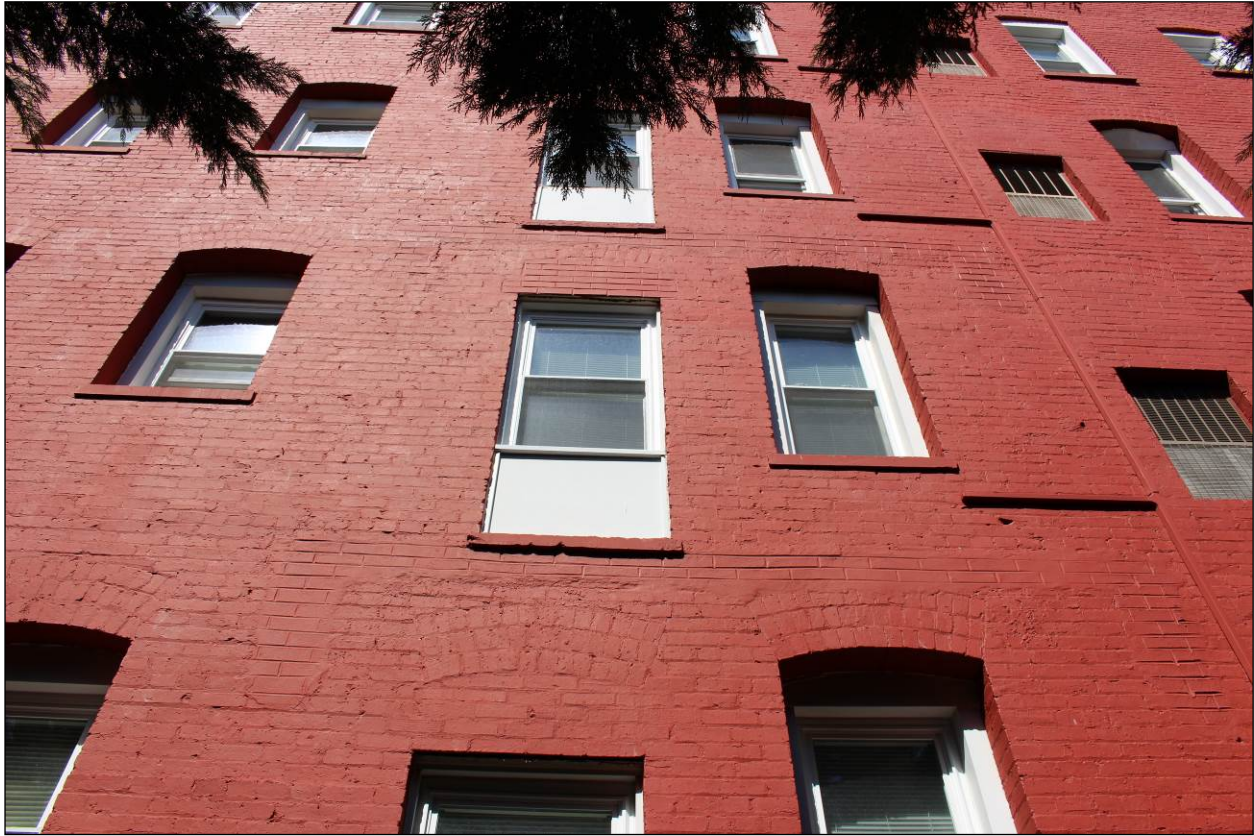
Exterior: Windows on south elevation, looking north
