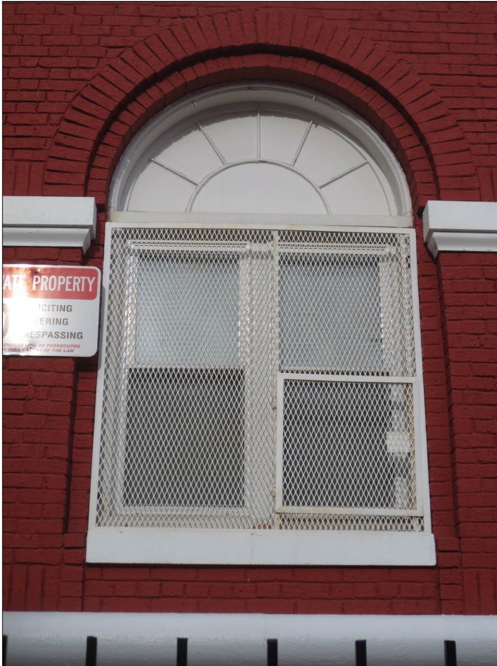
Exterior: Detail of first floor window on façade, looking west
