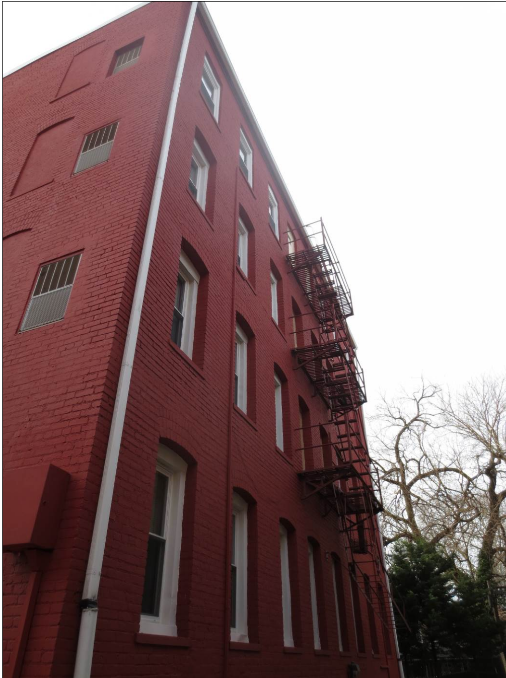
Exterior: Rear (west) elevation, looking southeast
