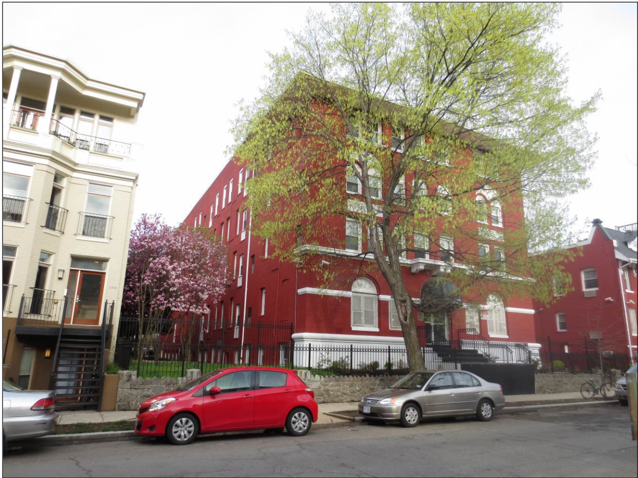
Exterior: Façade and south elevation, looking northwest
