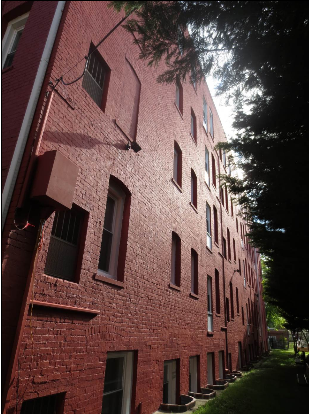
Exterior: South elevation, looking northeast
