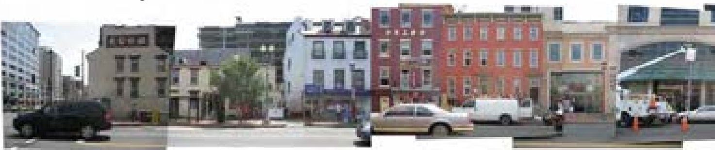
600 block of H street, looking south
