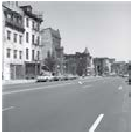
General view northeast down H Street NW from 9th Street. To 7th Street, the Chinatown Friendship Archway, 1987
