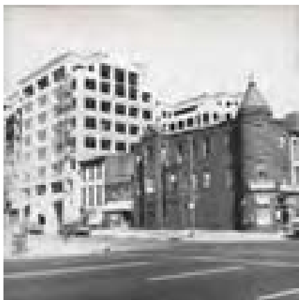
General view northeast down 8th Street NW from H Street. Office building construction, 1991
