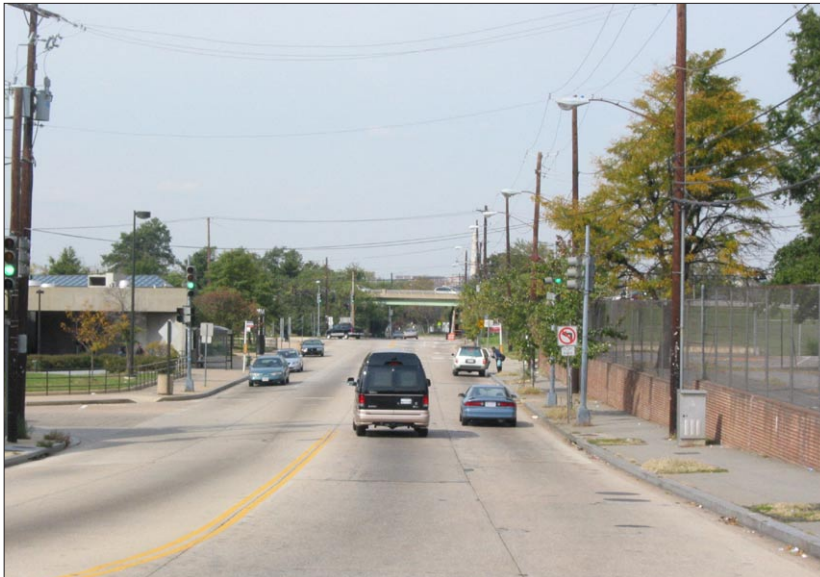
View down Howard Road along the Metro Station
