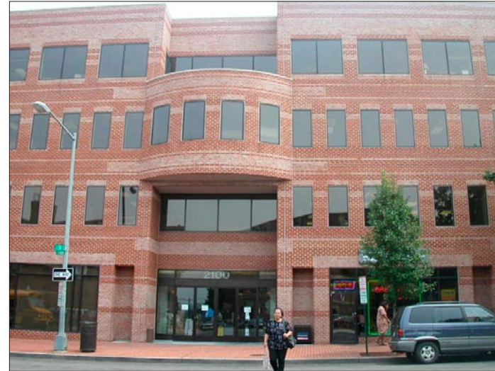
Existing office building along MLK
