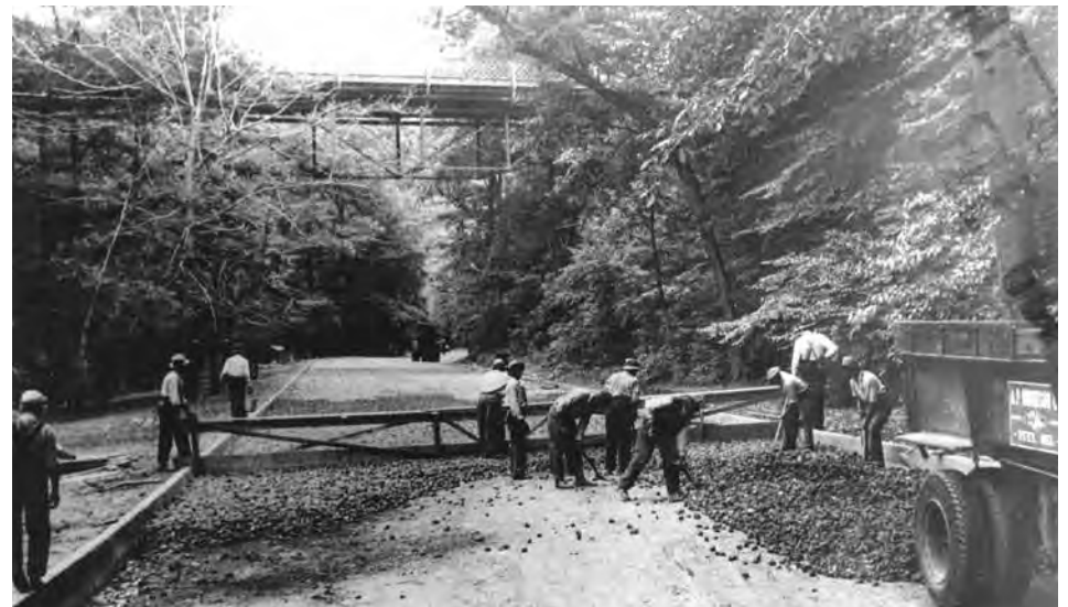
PWA workers building Piney Branch Parkway
